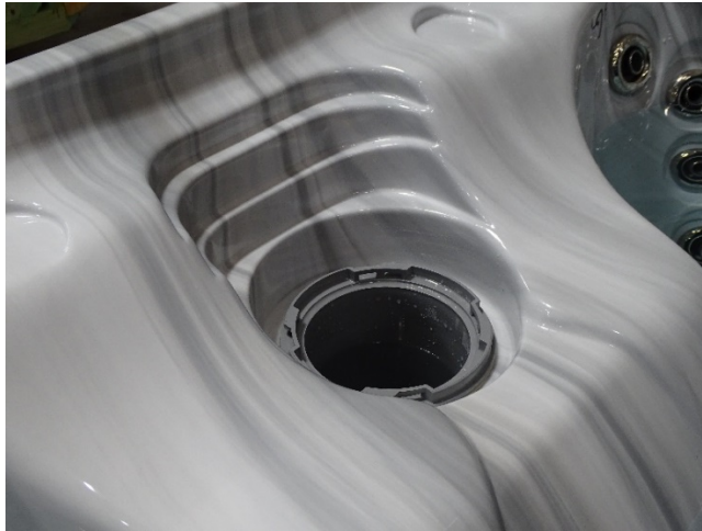
Figure 45. Empty filter housing
